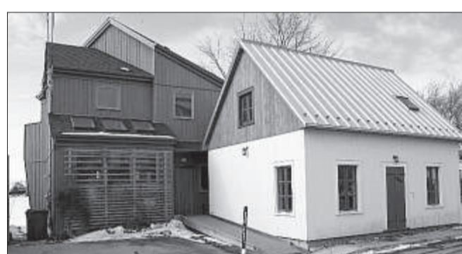
Plumb restored the original structure, at right, and then added a new one to the back of the property.
